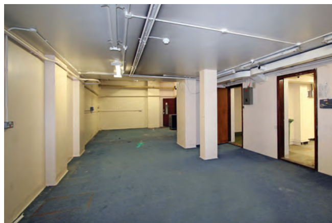
All the rooms in the Emergency Centre are now stripped of all fixtures and fittings although ventilation trunking can still be seen in all the rooms
